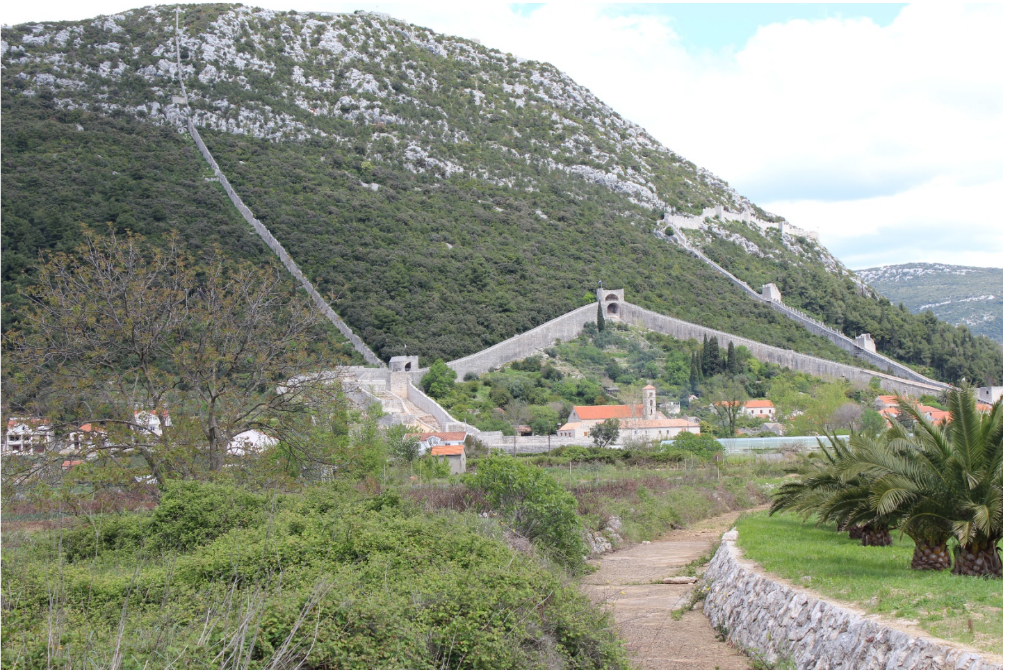
The old walls of Ston
